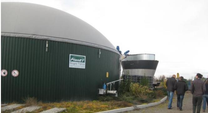
Pilot projects (see [www.combine-nwe.eu](http://www.combine-nwe.eu)) are being set up in the UK for small scale combined heat and power, using experience from similar plants in France and Belgium. Biomass is separated into cake which can be dried and pelleted as solid fuel, and fluid which can be fermented into biogas which can produce thermal and electrical energy.
