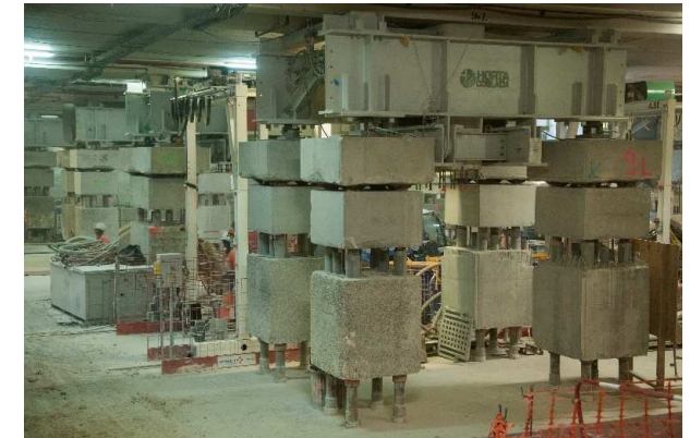
1.E) Excavation and completion of the underpinning
