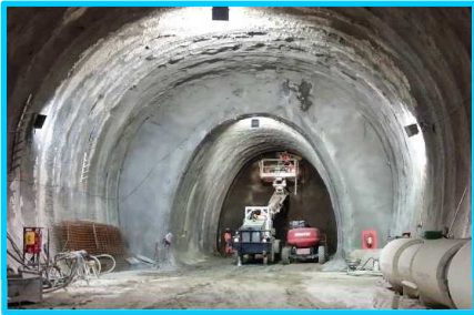
EXCAVATION FOR THE CENTRAL PILLAR – EASTBOUND CAVERN
