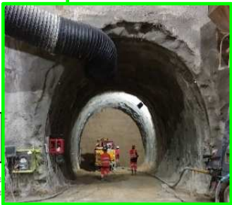
EXCAVATION FOR THE CENTRAL PILLAR – EASTBOUND CAVERN
