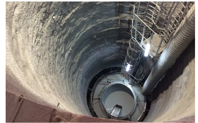
1.J) Construction of the “elephant foot” shaped base of the pillar
