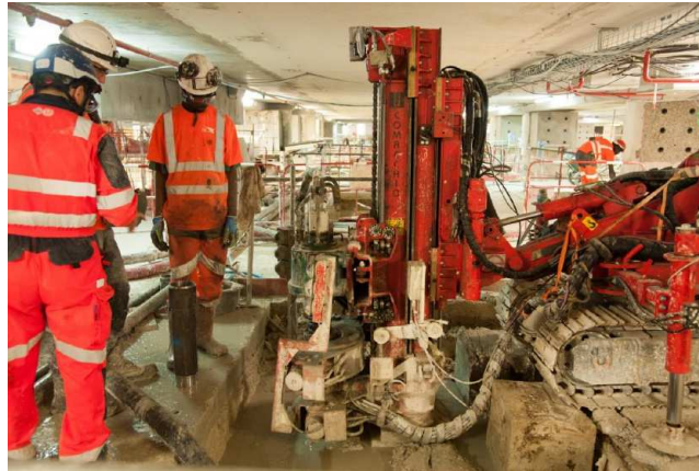
1.B) Execution of micropiling (15 km)
