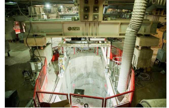
1.H) Installation of gantries and easements within the shafts
