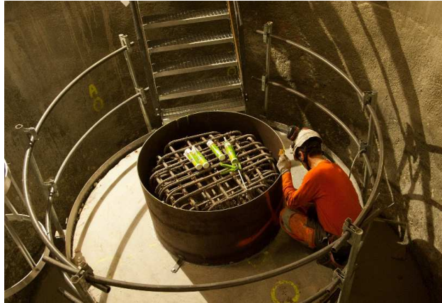
1.K) Climbing formwork in 3m lifts for the realisation of the reinforced concrete final pillars
