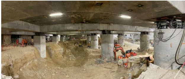
2.D) Excavation of the “cathedral” part of the mega-station under the transfer slab
