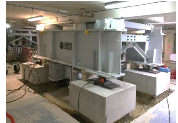
1.C) Steel bearing structure on micropiles, tightened to each existing column. Jacking of the existing structure and separation of the columns from their old footings
