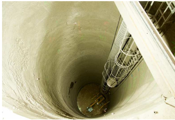
1.I) Excavation of the 22m deep pillar shafts by steps of 1.0 m to 1.2 m, then lining top-down
