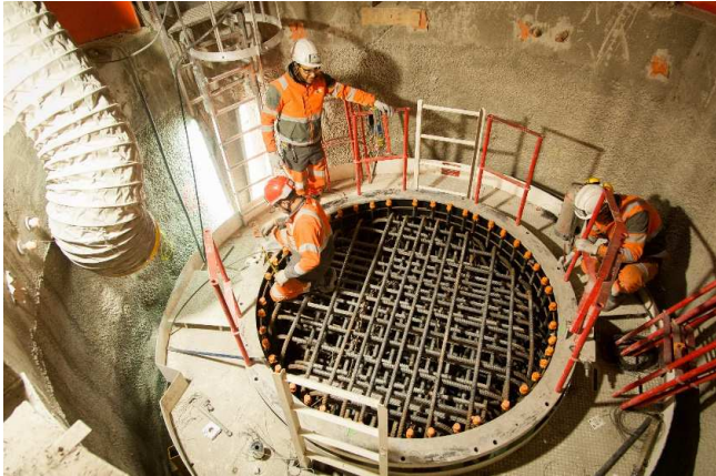
1.K) Climbing formwork in 3m lifts for the realisation of the reinforced concrete final pillars
