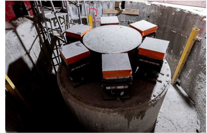
1.L) Installation of jacks on the head of each pillar: 6 to 8 jacks per pillar, total transfer capacity 100 000 ton
