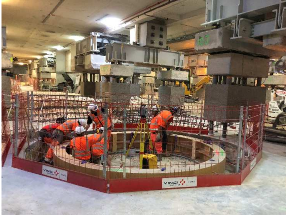
1.F) Paving and shafts' capping beams
