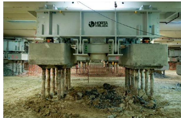
1.D) Excavation and hydro-demolition of the old foundation footings
