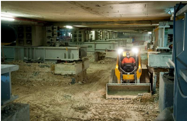
1.D) Excavation and hydro-demolition of the old foundation footings
