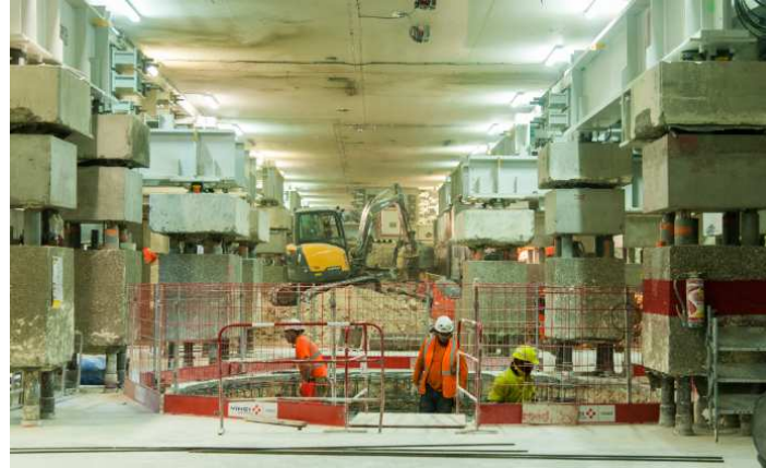
1.G) Execution of the 60+1 shafts for the 60 pillars and the site logistic
