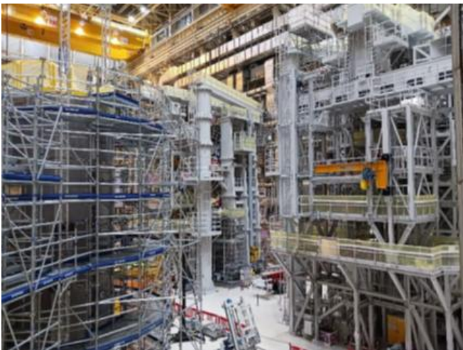
Assembly Hall with gantry crane
