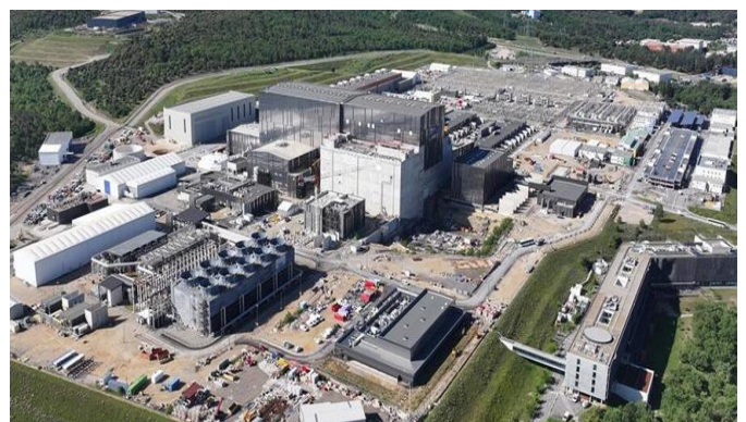
ITER Site with Tokamak Complex & Assembly Hall
